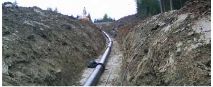
Deflectable by up to 5°, which saves time and fittings
